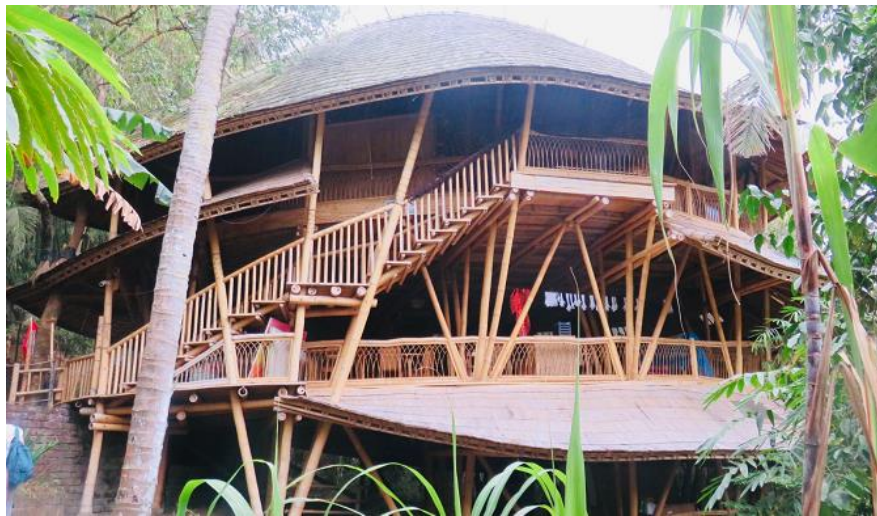
Fig.7 the bamboo construction
